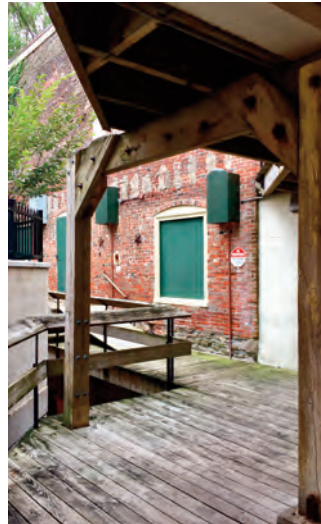
Palmer's Bakehouse still stands tucked behind the stores on S. 2nd Street.
